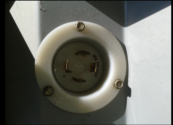
120/240 inlet plug on outside wall
