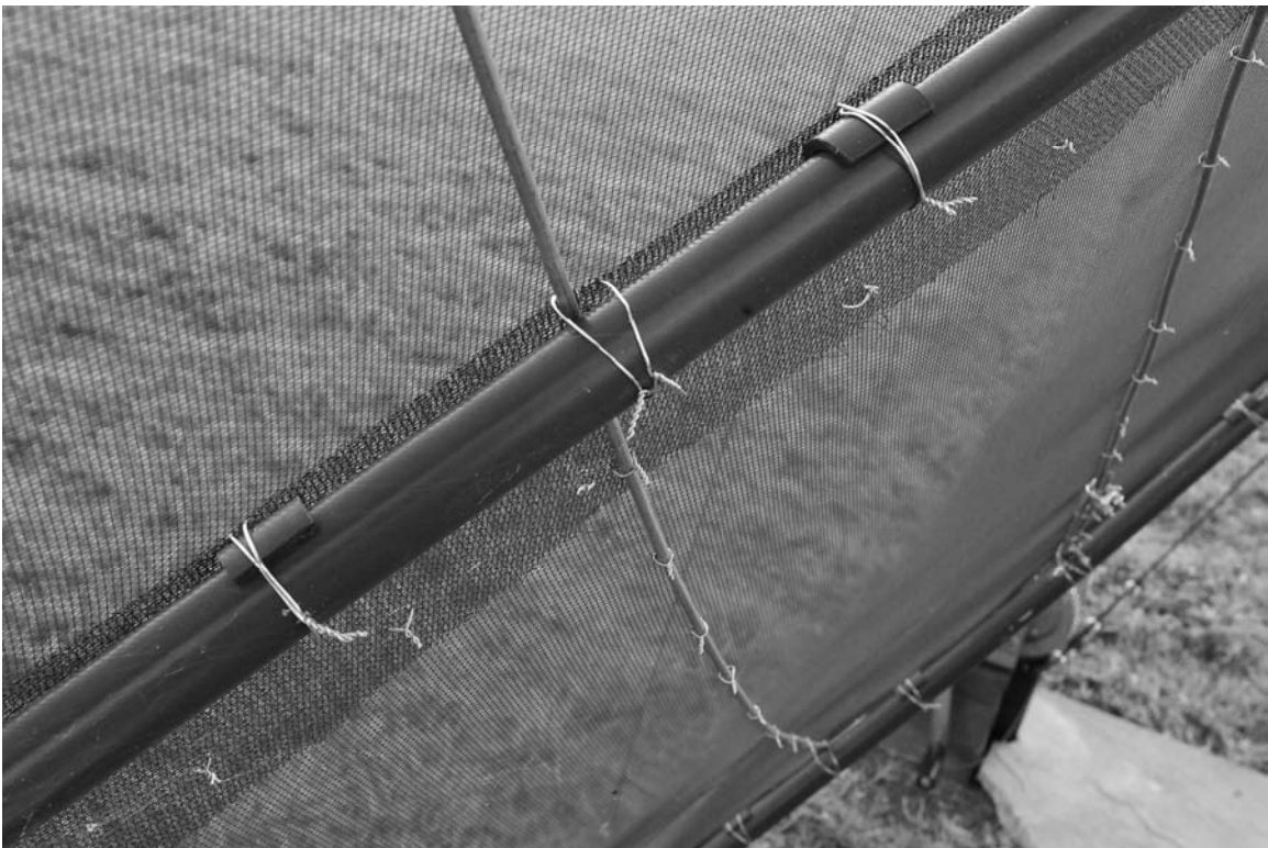
Fig. 12 – View of the mesh attachment method using aluminum MIG wire.
