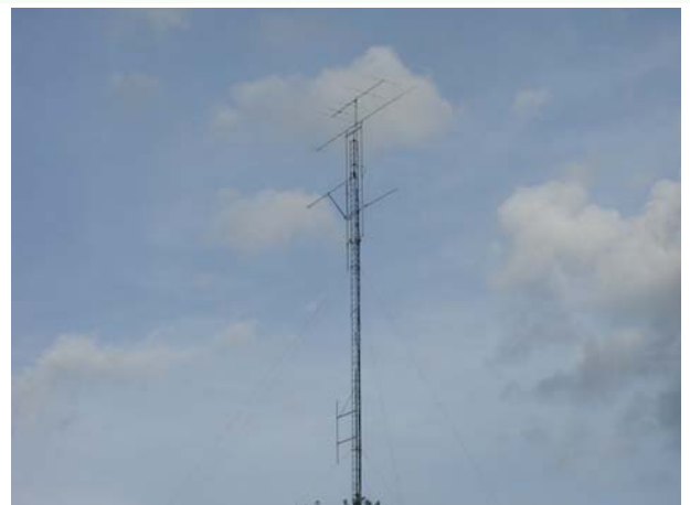
The pictures are taken at my contest location in FN01, It is a hilltop in the Allegheny Mountain range 2400 ft ASL. The tower is 155 ft of Rohn 55. It is located in the extreme NE corner of FN01, a stone's throw from FN02, FN12, and FN11
