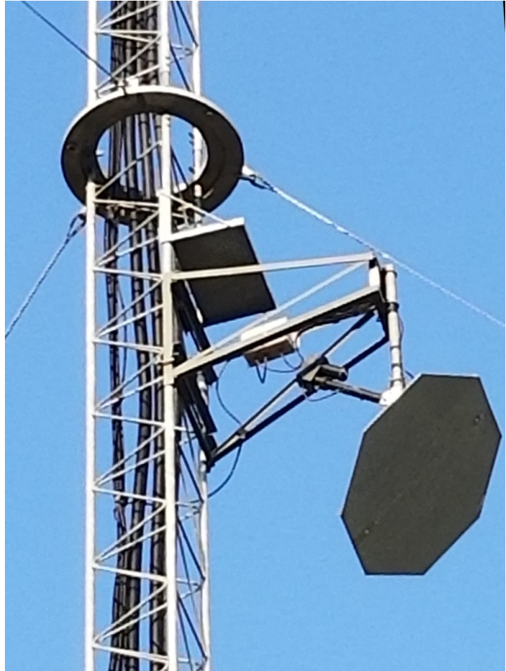
Figure 2 – W5LUA Flyswatter on rotating tower
